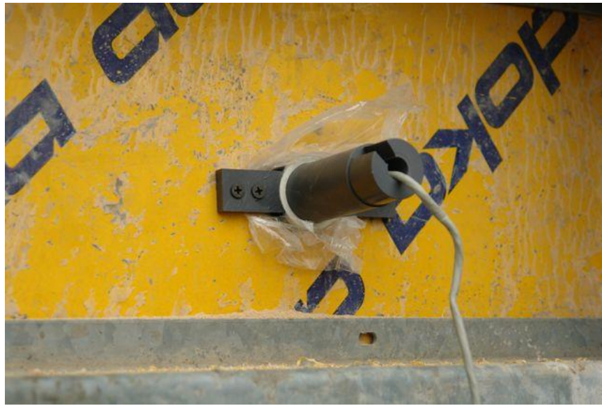
Figure 3 —Bracket with Pressure Transducer Attached to Formwork
